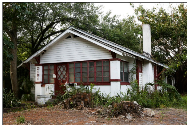
Figure 1: The structure at 2101 3 rd Ave N before it was condemned and demolished in 2018.
